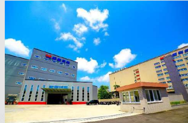
Chansing Factory II Server System Integration Factory
