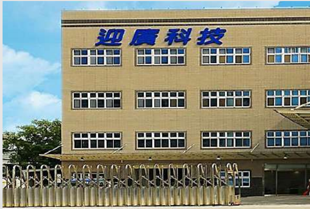
HQ Server System Integration Factory
